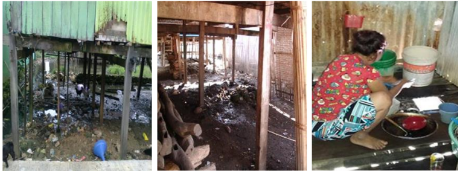
Figure 8. Drainage of the house on stilts directly throw to the kolong and the form of grey water disposal from the service area on stilt houses
