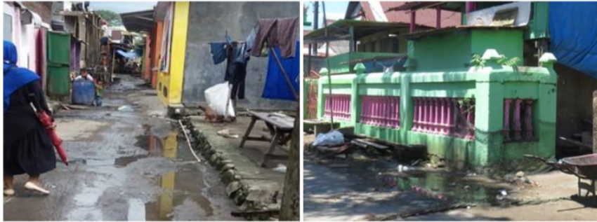
Figure 5. Street drainage condition in residential environment
