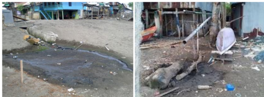
Figure 4. Drainage in coastal area
